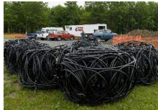
Geothermal slinky loops await installation at Red Tail Ridge Winery in Penn Yan. (Provided photo)
